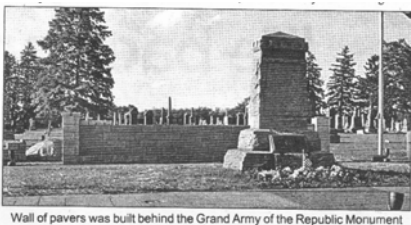
Wall of pavers was built behind the Grand Army of the Republic Monument
